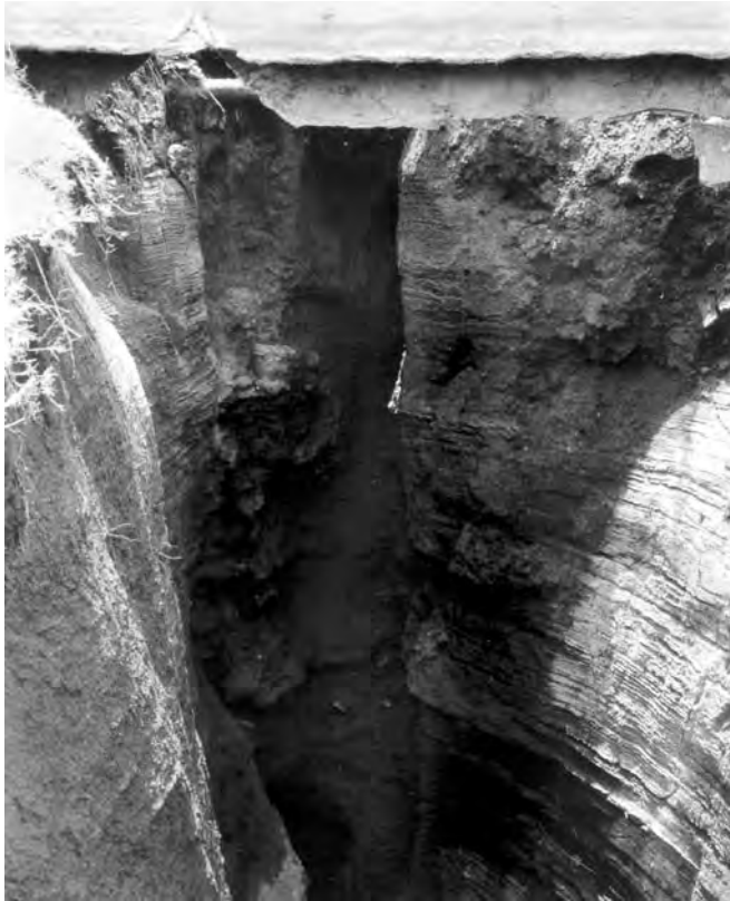
Figure 12.9. A concrete foundation, directly on dolomite bedrock in South Africa, that has retained integrity after an open fissure has been exposed beneath it when its soil fill was washed out.
