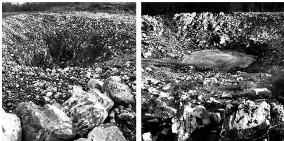
Figure 12.5. Solution sinkholes exposed during construction along a highway footprint in Slovenia, one cleaned out ready for filling, the other with a concrete plug forming its floor. Photos: John Gunn.
