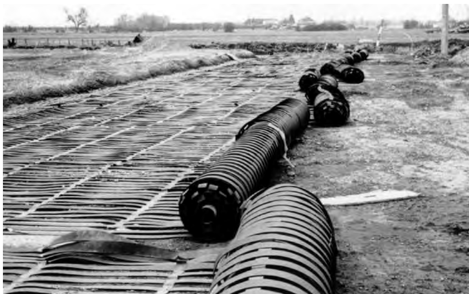
Figure 12.7. Heavy paralink geogrid being rolled out onto a road sub-base as a protection measure against sinkhole development in the underlying soil.
