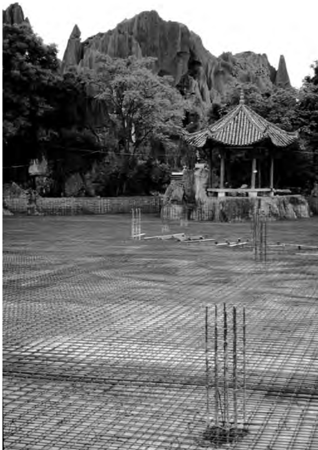
Figure 12.2. Double weldmesh reinforcement for a concrete slab, cast as foundations for an ornamental lake with a bridge and pagoda, on deep soils over pinnacle karst at Shilin, southern China.
