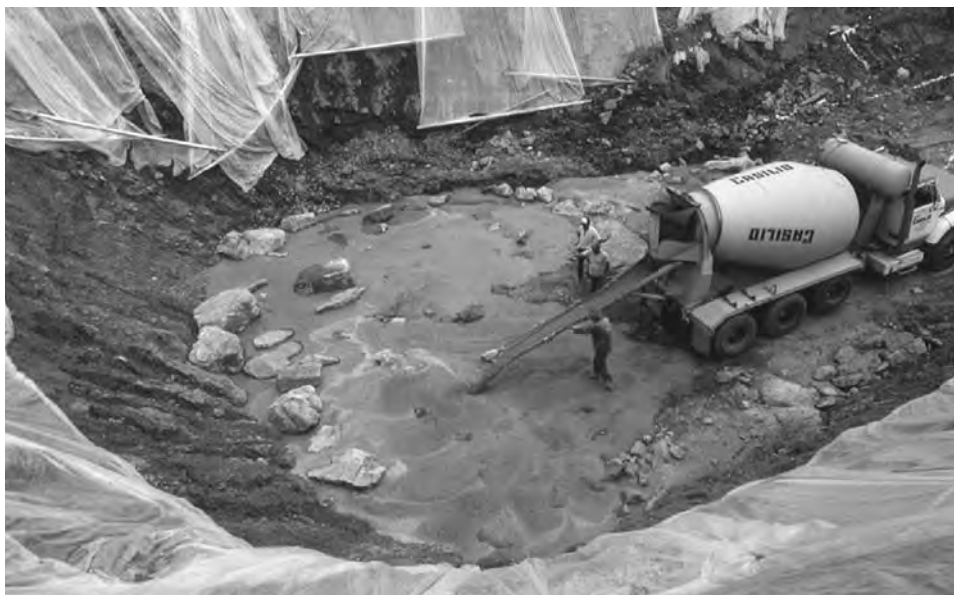
Figure 11.10. Pouring the last of the concrete into the plug of chunk rock in the Macungie sinkhole, before rebar was laid as reinforcement to a cast concrete cap.
