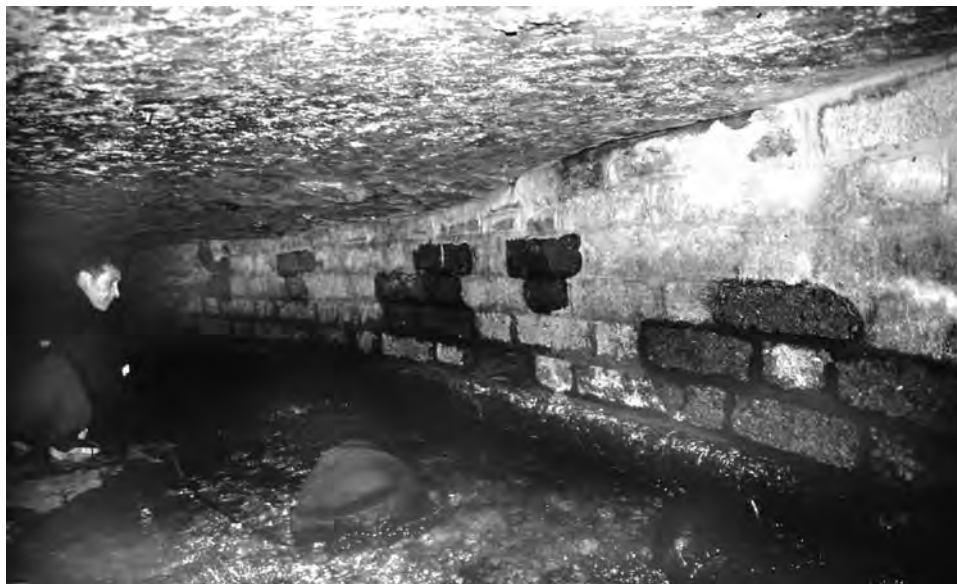
Figure 12.13. A masonry wall built beside the underground stream inside the St. Augustine's Cave in Ireland in order to reduce the unsupported span beneath a main road that stands on a concrete slab.
